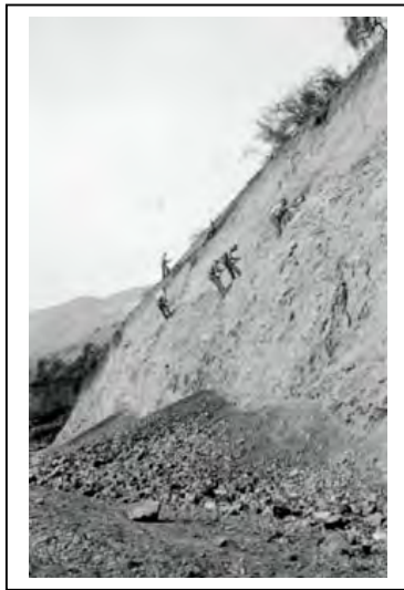
Figure 12: Convict labor cutting slopes in 1932 during construction of the Carmel-San Simeon Highway.
