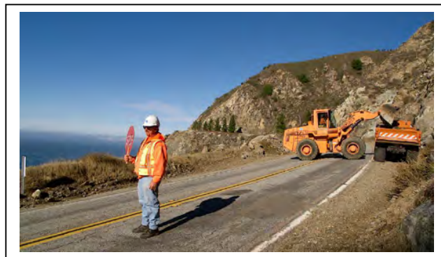
Figure 25: Road crew working to remove material from a landslide
