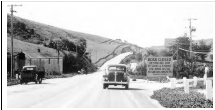
Figure 22: The corridor has suffered landslide-related closures ever since the highway's opening in 1937.
