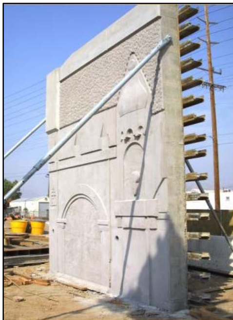
Test panels serve as a benchmark for measuring consistency and controlling the quality of the wall structure aesthetic treatments.
