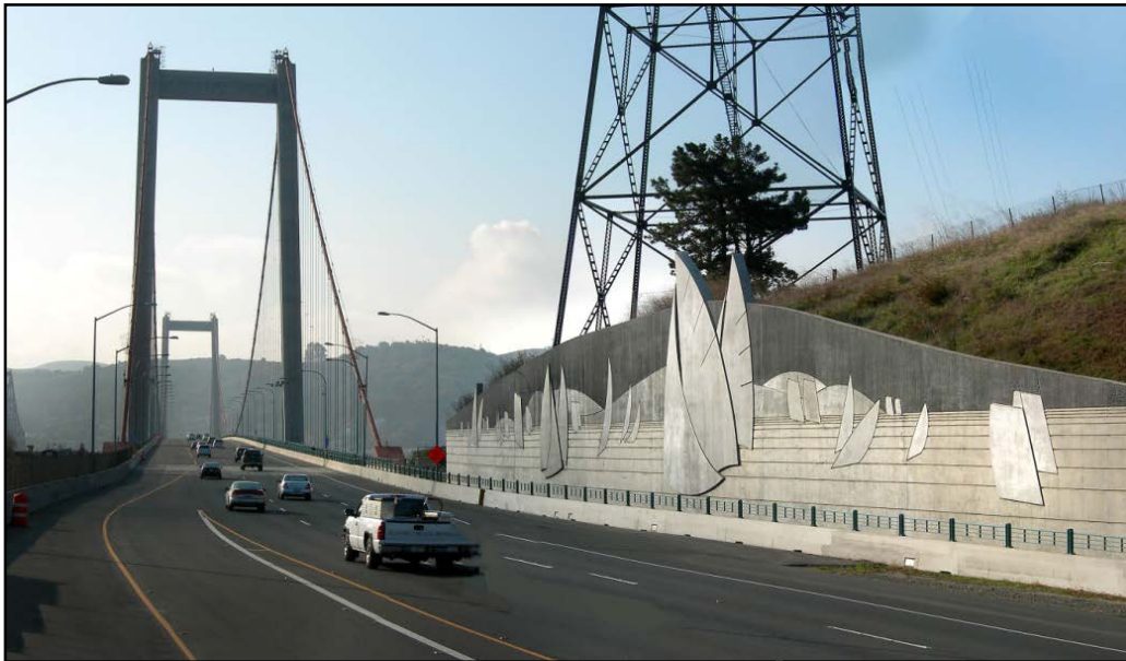
Aesthetic treatments on wall structures can reflect an image of the surrounding community and create visual interest for motorists.
