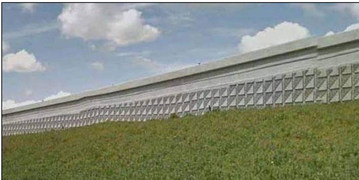
The staggered appearance and misaligned pattern of this wall structure are the result of inadequate coordination of the aesthetic design, wall design, and construction methods.
