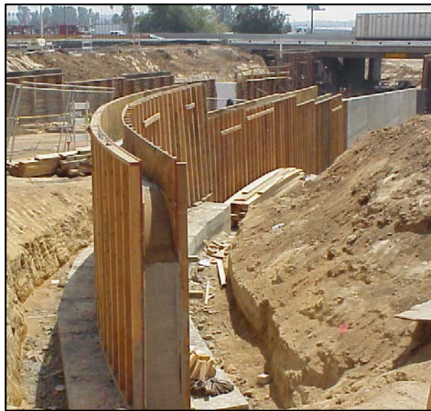
Gang form systems are the common methodology for wall structure construction.
