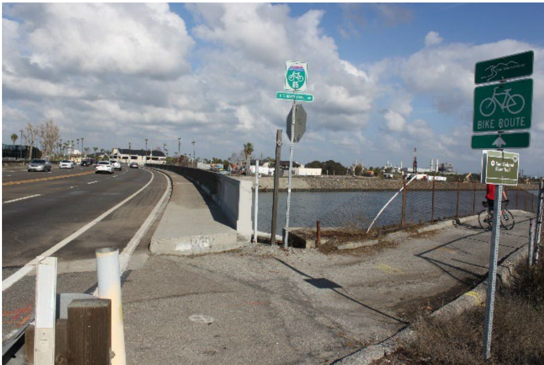
Figure 3 View of project area passing over bike path, looking north along SR-1
