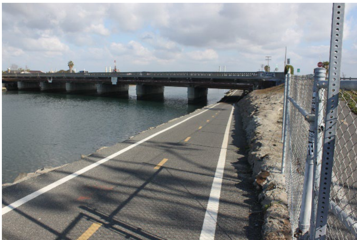
Figure 5 View of the bike path crossing under SR-1 looking east
