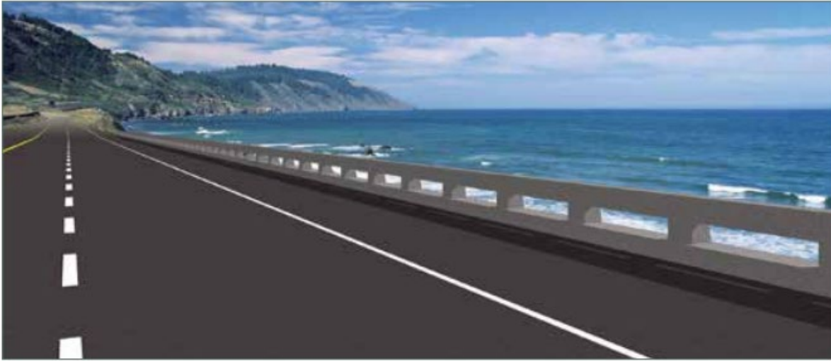
Figure 1.5-5 Concrete Barrier Type 80
