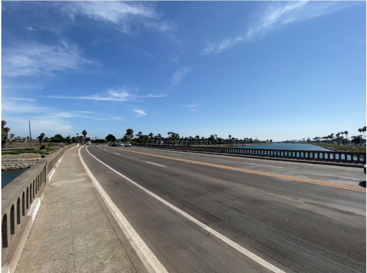
Figure 2.1-11 View looking southwest with an existing bike lane and traffic lanes with San Gabriel River
