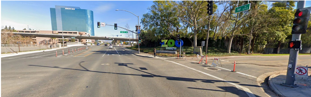
Figure 3. KEY VIEW (KV) #2 – From the Santa Ana Zoo and East 1st Street looking east. The existing I-5 elevated lanes are visible in the foreground. (The existing main I-5 lanes are below grade and not visible.)
