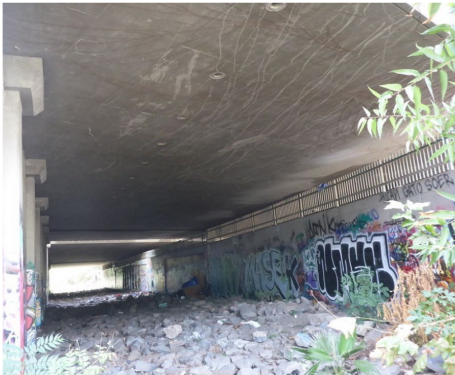
Figure 2-4 Bridge Over Santiago Creek (55-1046R) Looking Downstream
