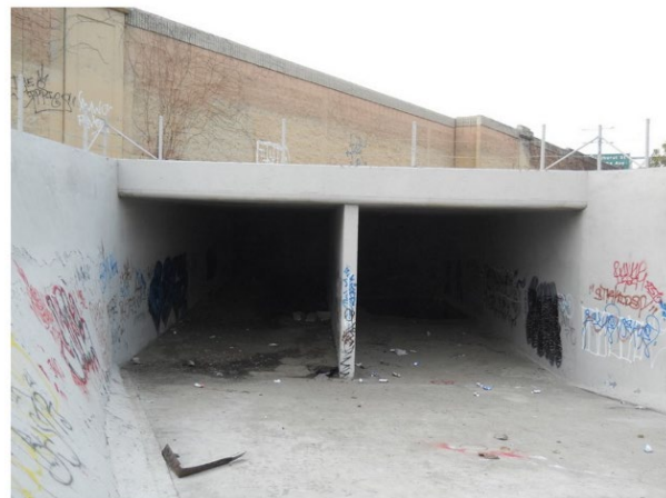
Figure 2-2 Bridge Over Carbon Creek (55-0910) Looking Downstream
