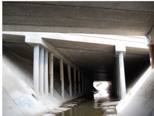
Figure 2-1 Bridge Over Fullerton Creek (55-0087) Looking Downstream
