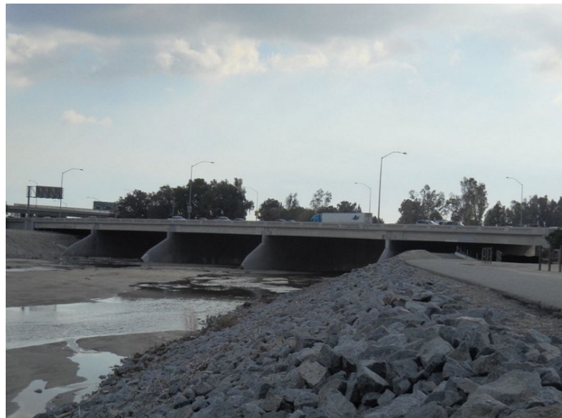
Figure 2-3 Bridge Over Santa Ana River (55-0811) Looking Downstream
