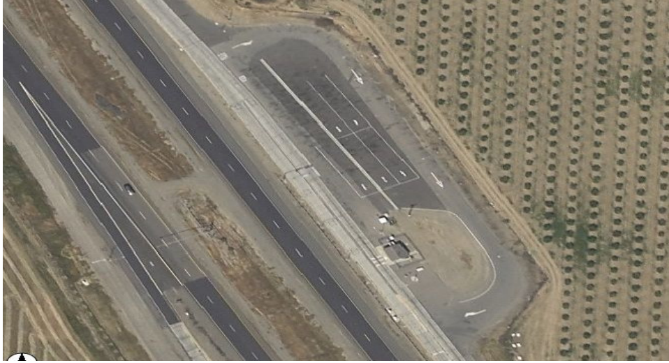
Class "C" Facility at Santa Nella, CA
