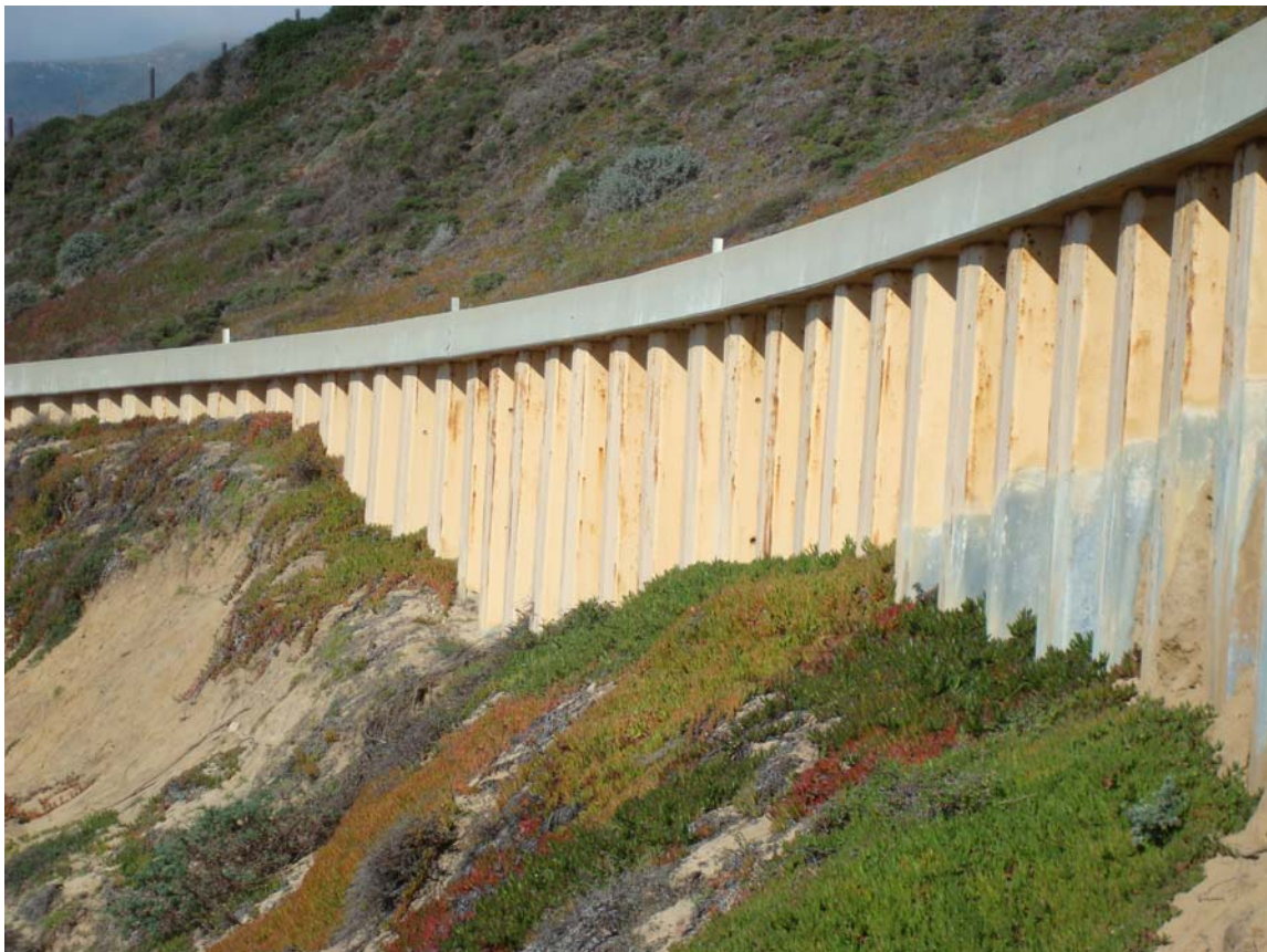
Figure 6-1. Sheet Pile Wall with Cap Beam
