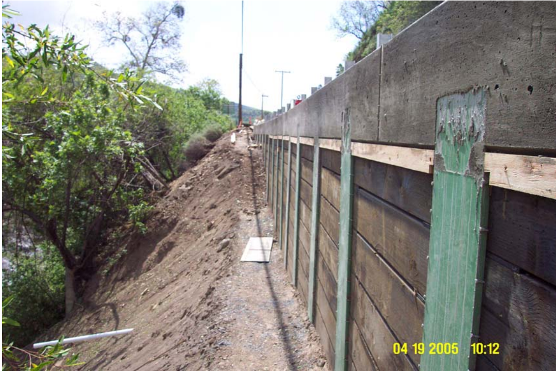
Figure 6-2. Soldier Pile Wall with Cap Beam
