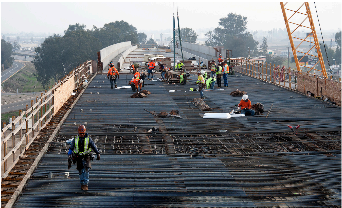
Workers supporting high speed rail construction in Fresno
